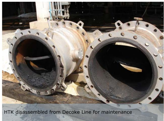
HTK disassembled from Decoke Line for maintenance
